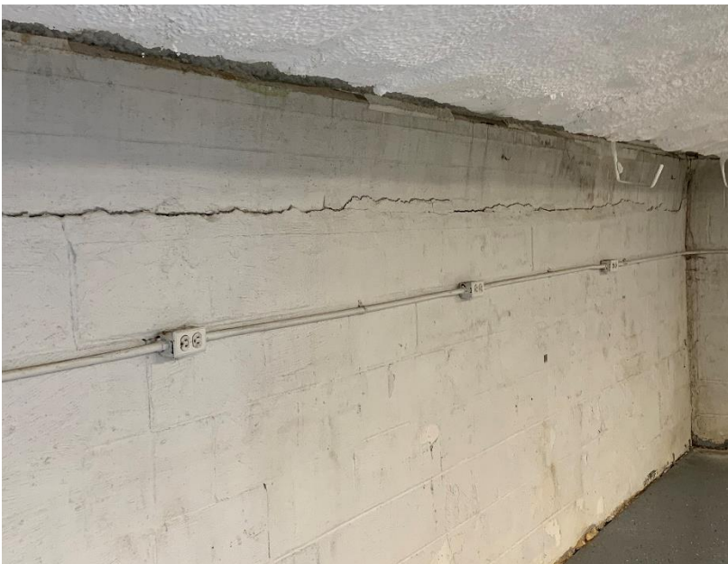
Cracking along the length of the top of the skirt wall along the front of the Home side bleachers.
