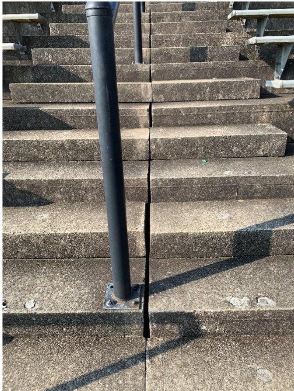
Absence of joint sealant between concrete planks.
