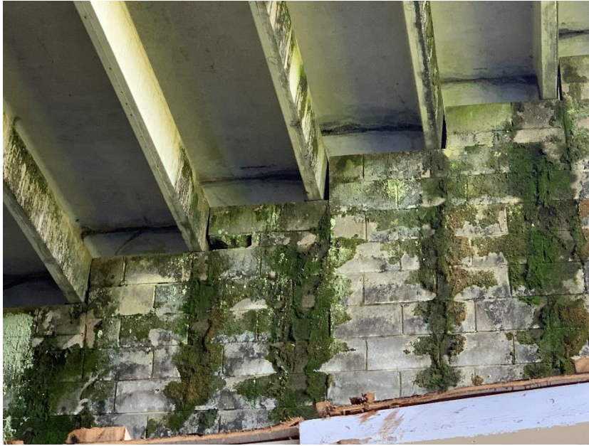
Water infiltration, moss growth, cracking and loss of section in interior masonry wall.
