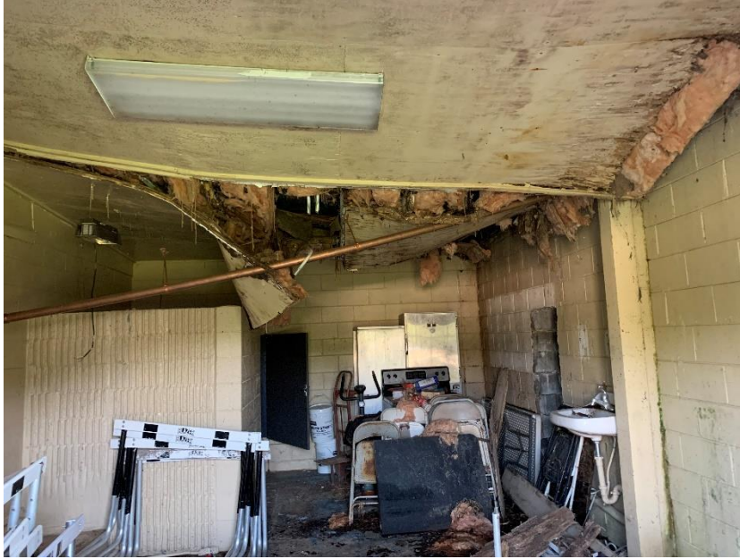
Water infiltration to built-out area beneath bleachers.
